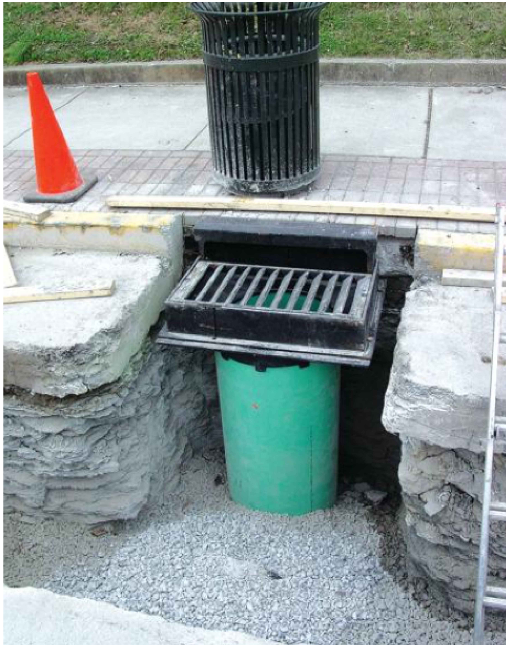
TYPICAL NYLOPLAST ROAD INLET
