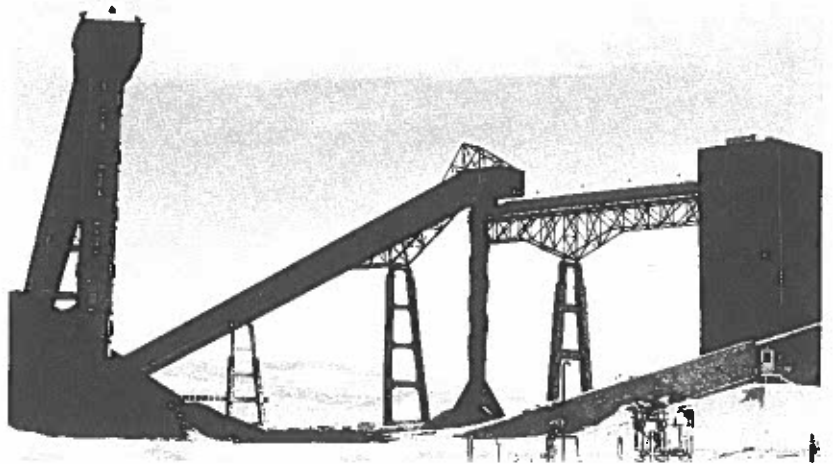
At Colorado-Ute's coal-fired power plant.
